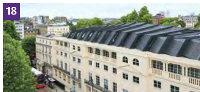
Which? Headquarters – Offices
