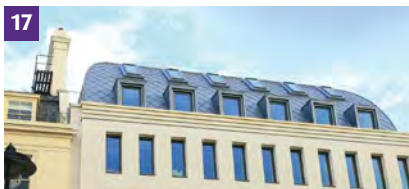
73 Brook Street – Offices
